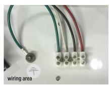
Connect power supply leads to terminal block (if supplied) or directly to the black and white driver box.
