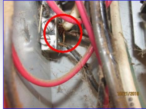
*Double tap and frayed wires not fully connected to bus bar*
