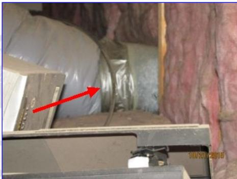
*Duct tape used to seal duct.*
