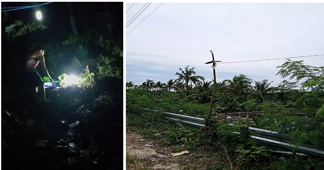
Figure 11. Two Bulb Generated Power and Constructed Street Lighting Post
