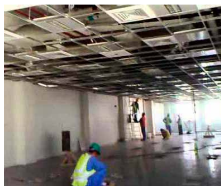
Ceiling works (Cables-fire protection-AC-lights)
