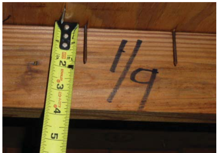
#3 ROOF DECK ATTACHMENT 8d NAILS
