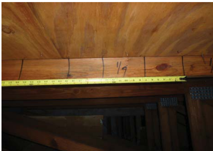
#3 ROOF DECK ATTACHMENT 6" X 6" NAIL SPACING
