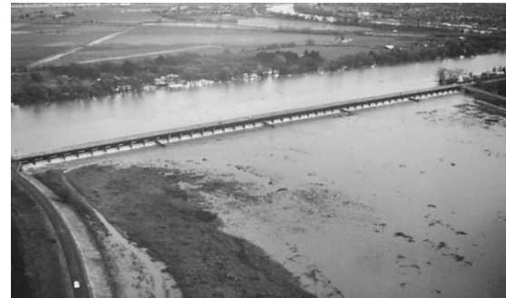
Sacramento Weir (one of five major State Plan of Flood Control weirs) as it appeared during the 1995 flood. The weir opens to release flood flows.
