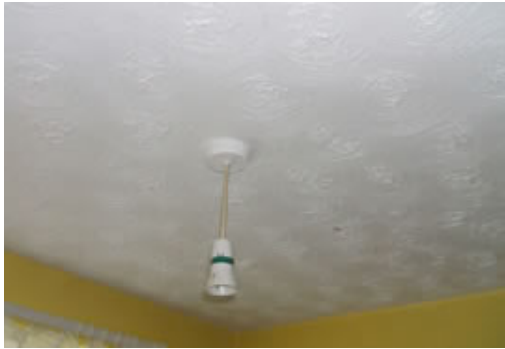
Asbestos textured coating
