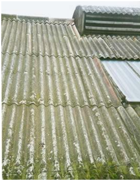
Asbestos cement roofing
