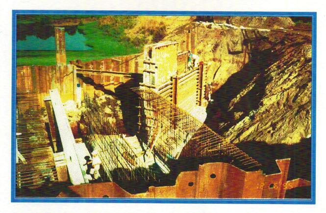
Construction management and on-site inspection services were performed by Constructioneer Corporation for this project consisting of bridge demolition and bridge/roadway construction. The project allows for roadway widening and corrects the scouring and undermining that was existing with the original structure due to the inadequate depth of the base of the culvert.
