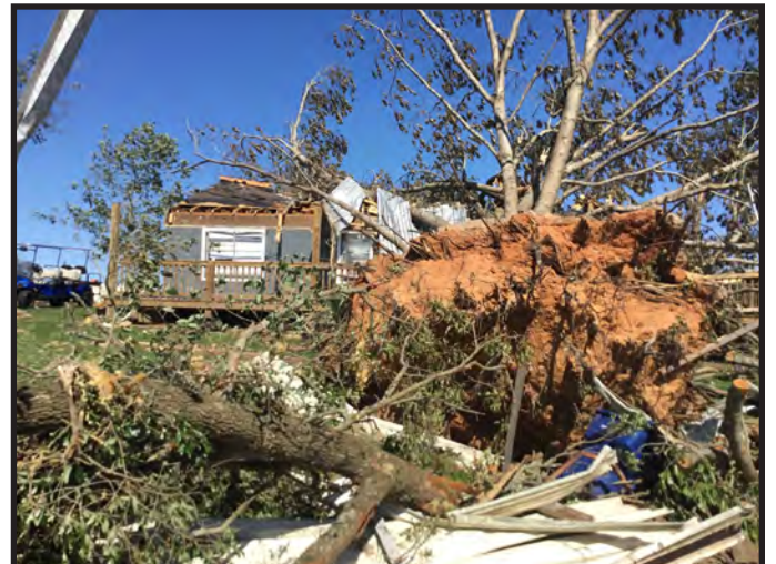
Tornado damage, Onalaska, April 2020. Photo credit: NWS.
