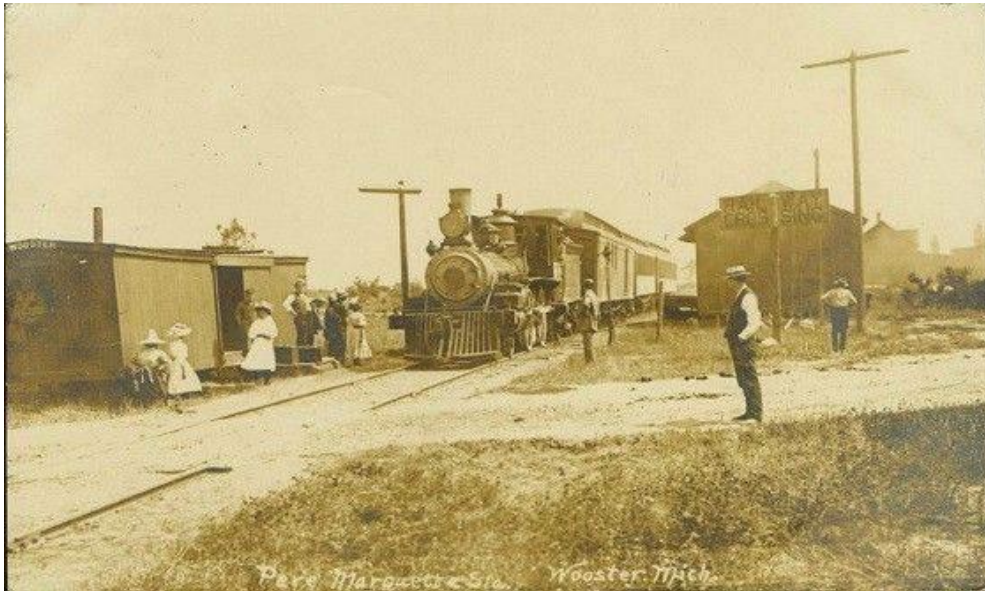
Wooster Railroad Depot and Post Office
