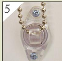
5 Using screws provided, install tension device with the maximum tension on the loop while still allowing ease of operation
