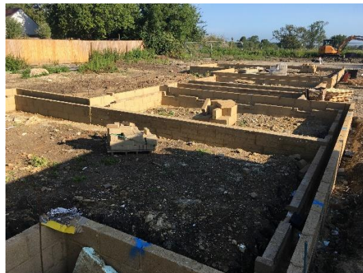
Block work below DPC to plots 7 and 8.
