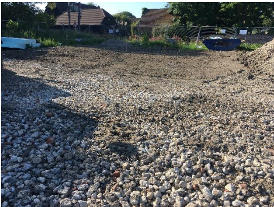
Plots 1 and 2 cleared ready for foundations.
