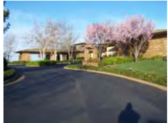
Entrance Drive Asphalt Pavement
