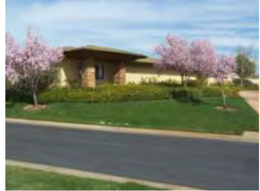
Exterior Surfaces - Typical
