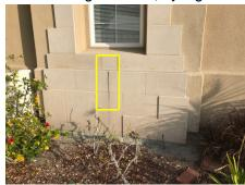
**44:** Siding water damage. Unable to tell if there is additional hidden damage behind the siding. Recommend further evaluation / repair or replacement of all siding to keep moisture and insects from harming structure by a general contractor.
