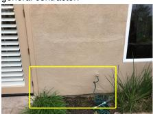
**45:** Water from the roof is staining the siding. This is due to the lack of a functional gutter system. This is a moisture intrusion hazard. Recommend installing gutters by a roofing contractor.
