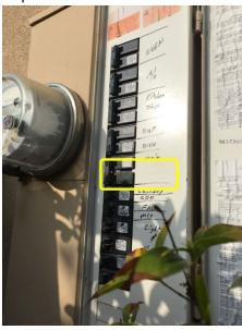
**86:** Panel cover screw missing. Panel cover should be secured to the panel. This is a shock hazard. These screws should be approved, flat tipped screws. Screws can be purchased at any home-improvement store.
