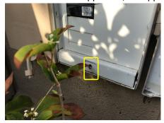
**87:** Access to electrical panel is blocked, there should be a 30" wide by 36" deep cleared area in front of the panel (all the way to the ground). Recommend you clear the area in front of the panel for safety purposes.
