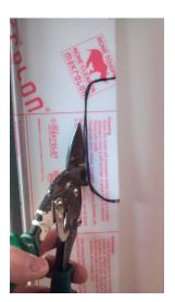
Step 4 – Mark and cut closure strips to fit around handrail, etc. using tin snips. Closure strips may be bent by hand or with duck bill pliers. Lap strips to make an air tight seal.
