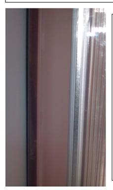
Step 6 – Compress the soft gasket material to the wall and apply the closure strip to the double sided tape. This will hold the closure strip in place and make an air tight seal.
