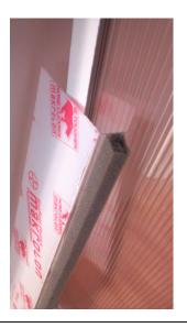
**Step 3** – Remove protective film from the edge of the closure strip and apply <sup>3</sup>/<sub>4</sub>" x <sup>3</sup>/<sub>4</sub>" soft foam gasket material.
