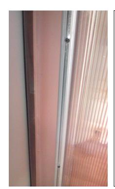
Step 7 – Install screws though the closure strip into the sheet metal strip. DO NOT SCREW INTO THE ALUMINUM.
