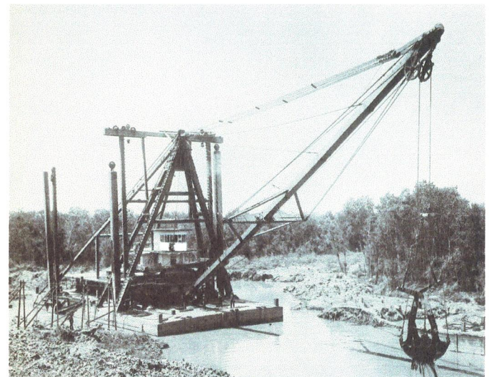
Clamshell Dredge built by Golden State and Miners Iron Works, San Francisco
