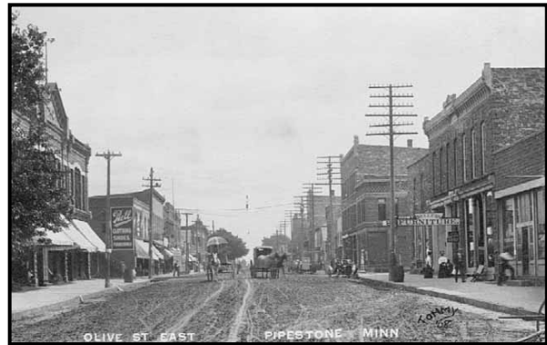
Olive Street East, Pipestone, MN (1908)
