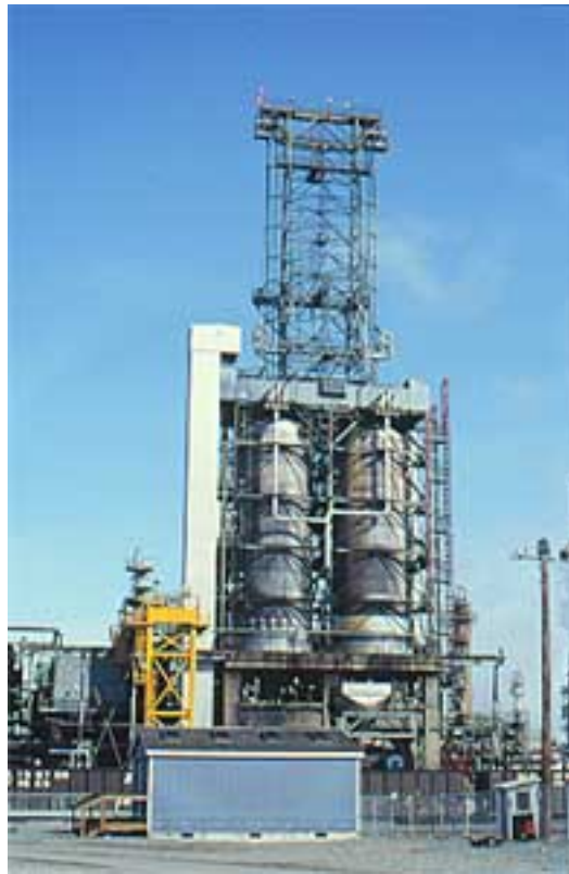
Delayed Coking Unit
