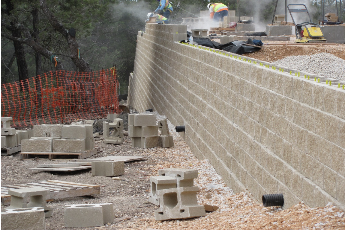
EXHIBIT 7 – RETAINING WALL CONSTRUCTION 12.18.20
