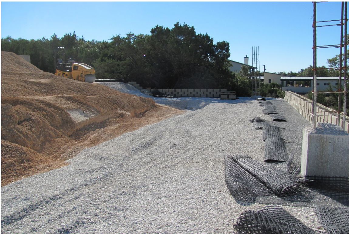
EXHIBIT 6 – RETAINING WALL CONSTRUCTION / GEO GRID 12.14.20
