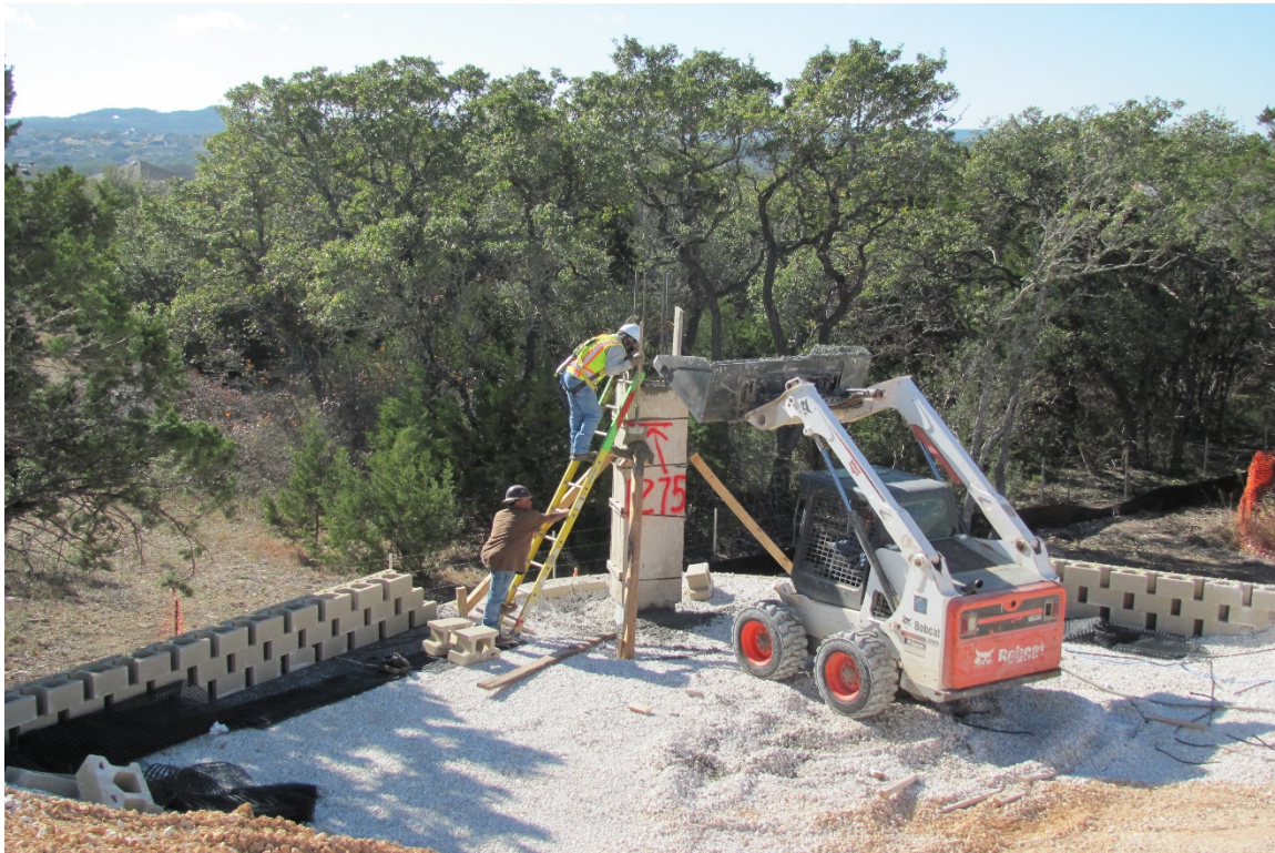
EXHIBIT 10 – RETAINING WALL / LIGHT TOWER CONSTRUCTION 12.23.20
