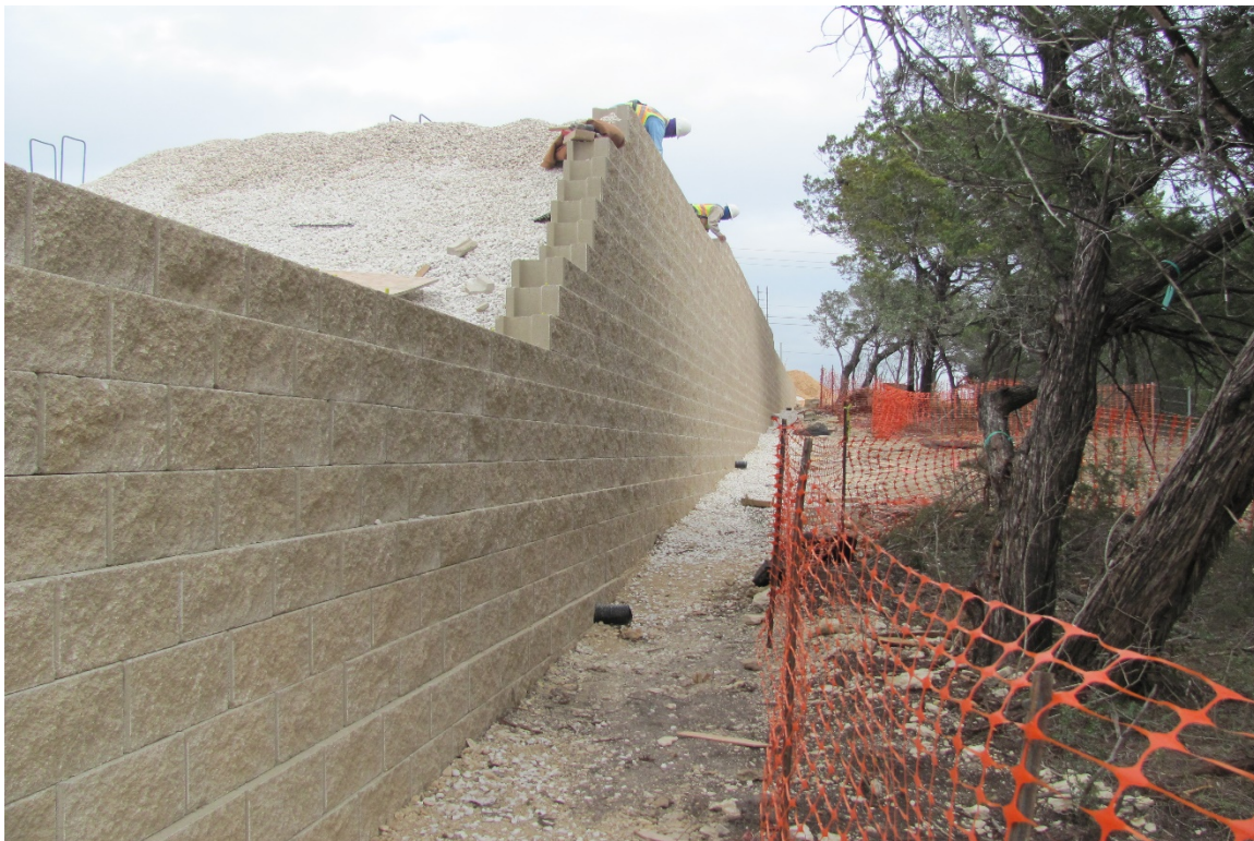
EXHIBIT 8 – RETAINING WALL CONSTRUCTION 12.18.20
