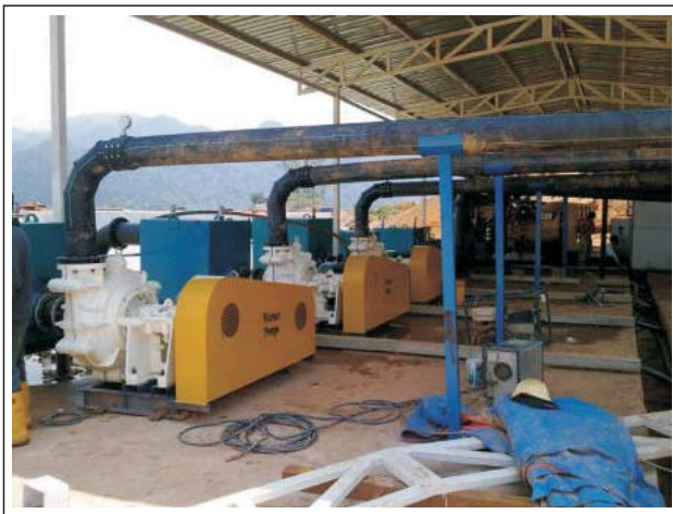
Thickener underflow pump in a copper mine 6x4D-WX Q=110m 3 /h, H=38m, n=1230rpm, \gamma =1.2
