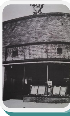
Early Times Office Building
