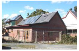
Buildings are mainly South facing in order to utilise Solar Gain to it's fullest. Under-floor Heating & Water Capture. Solar gain in area is 2.8 KWh per sq metre per day
