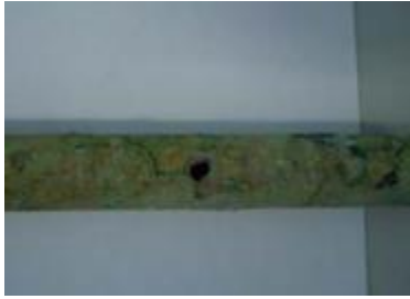
Figure 10: Copper Cracking and Corrosion (WSAA [6])
