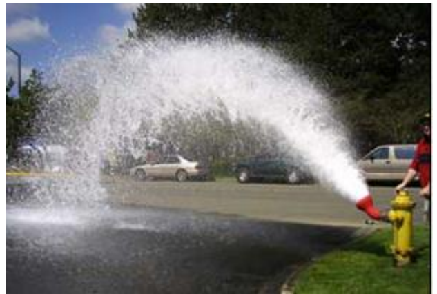
Figure 42: Annual Fire Hydrant Testing
