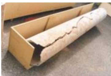
Figure 14: Asbestos Cement Cracking (WSAA [6])
