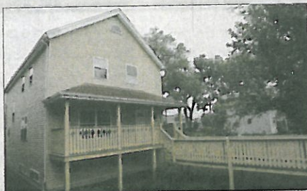
"Green" features in the Hurlock's home include carpeting made from recycled ketchup bottles and solar panels.
