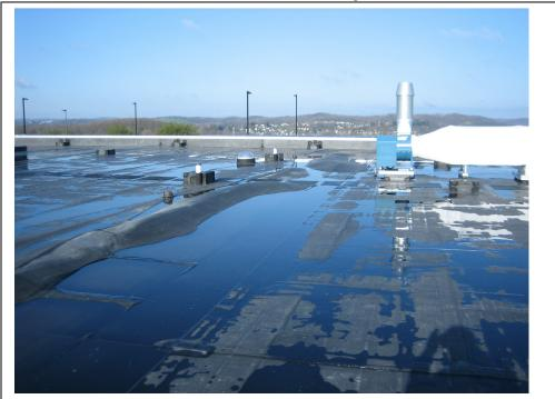
Photo 1 The photo demonstrates the typical condition of a recently installed fully adhered roof system over lightweight structural concrete. Bead adhesives were used to install insulation boards directly to the deck; no cover board was used.
