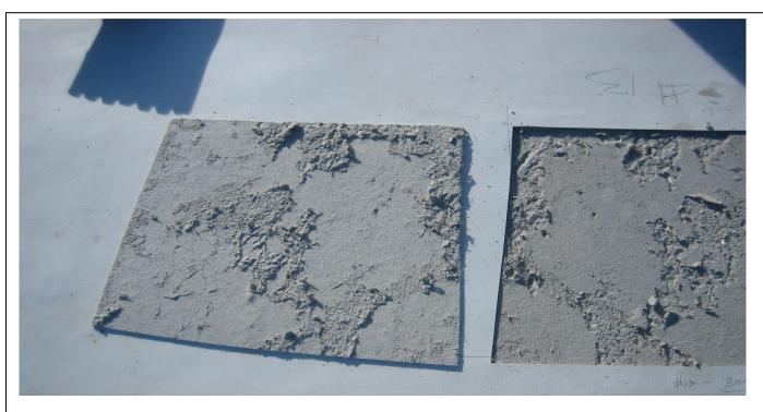
Photo 5 The new construction in a western state had a fully adhered roof system, white membrane and gypsum cover board. Moisture from the lightweight structural concrete deck drove up into roof system, wetting the cover board.
