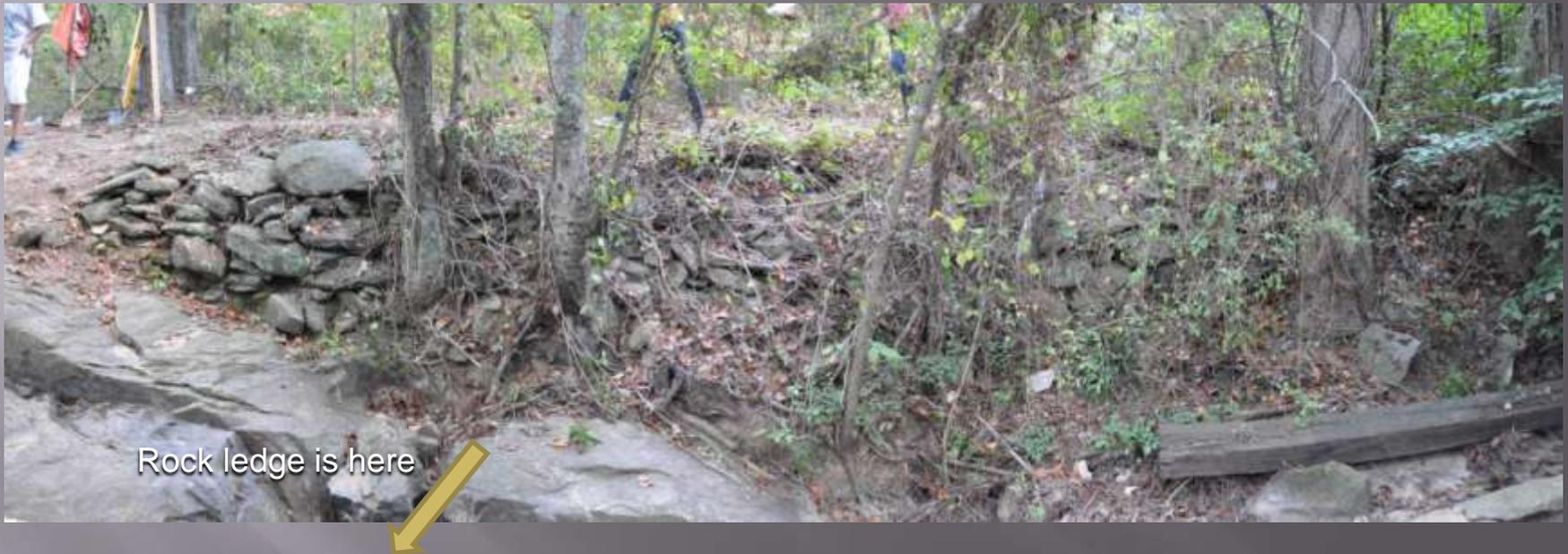
This is a fieldstone retaining wall for an old dirt road that parallels the stream on its east side. Only a portion of the wall, situated at and below the rock ledge, is shown here.
