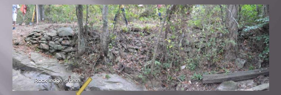
This is a fieldstone retaining wall for an old dirt road that parallels the stream on its east side. Only a portion of the wall, situated at and below the rock ledge, is shown here.
