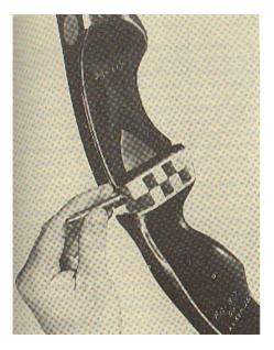
This is a detail of a Pearson Mercury Marauder Takedown Hunting Bow, This design just split the bow apart in the middle, using a locking pin to keep the bow together whilst shooting. This was not altogether successful, as wear in the joint was not good for accuracy and handle strength was reduced
