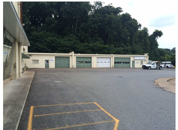
Side attached bays
