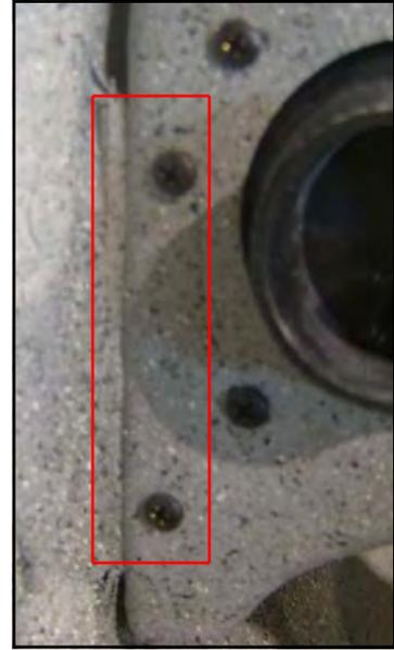
edge distance. You must determine the amount of overlap of the metal bracket and the panel box and drill on center.
