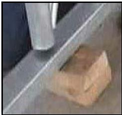
2. Begin by placing two 2x4 boards on top of each other at each end of the first curb. This will give you the approximate amount of spacing needed between the curb and the bottom of the stanchion. Refer to the Curb Measurement Chart for accurate measuring.
