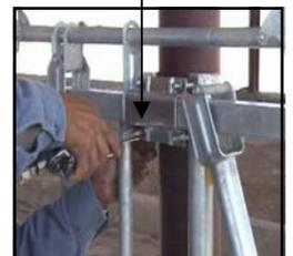
8. After you have loosely mounted each stanchion go back to the beginning of the "Run." You will now begin leveling the stanchions. Make sure that each stanchion is relative to the next stanchion and that both stanchions are leveled. Once the stanchion is level you can level and securely tighten the U-Bolts of the clamp.
