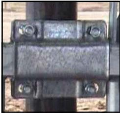
4. Place a clamp set around the Top Rail. Take a U-Bolt place it around the back of the post and through the top two holes of the clamp. Loosely tighten the clamp to the post and stanchion with the nuts provided. Place another U-Bolt around the back of the post and through the bottom two holes of the clamp. Loosely tighten the clamp to the post and stanchion with the nuts provided. Repeat this step for each clamp.
