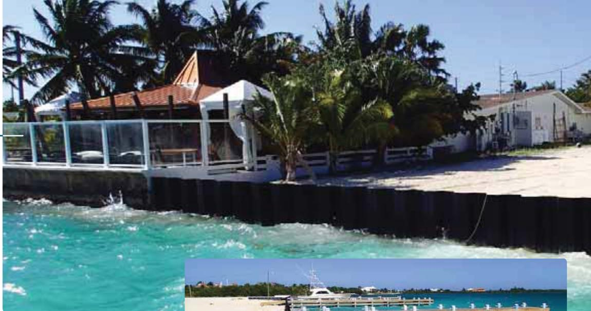
ing and the higher loading of axial roving results in a higher flexural modulus component that makes a PU pultrusion much stronger.” But Gulf’s hybrid PU pilings still exhibited less than *one-quarter* the MOE of steel pilings.
