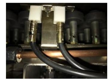
Remove old igniter and replace with new ignitor by reattaching all parts exactly as original model was setup
