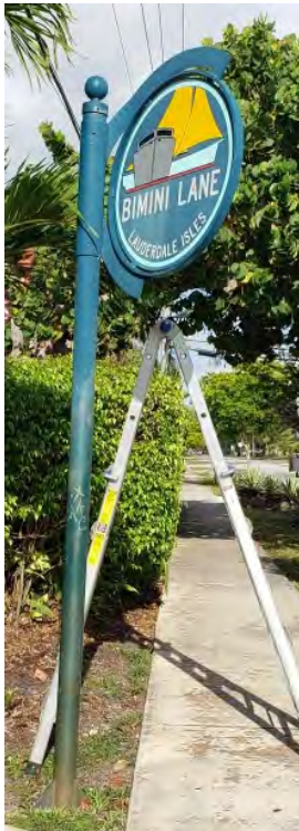
The Bimini Lane "before." Apparently the sign took a good hit from a truck cutting the corner— or maybe from one of the road crew machines.
