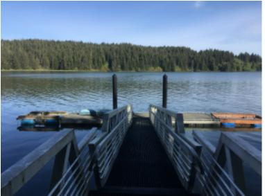
The floats supporting an old wooden dock started to deteriorate, so we replaced the deck and ramps with state-of-the art deck and ramps made from marine grade aluminum. We obtained Army Corps of Engineers approval, and the major renovation was completed in 2017.
