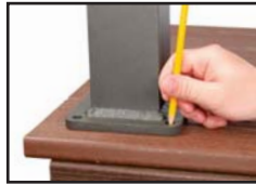
Mark and Pre-drill Holes
