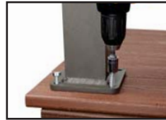
Fasten Post to Deck Surface
