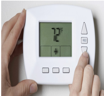
Step6 Turn thermostat off & on to ensure working
