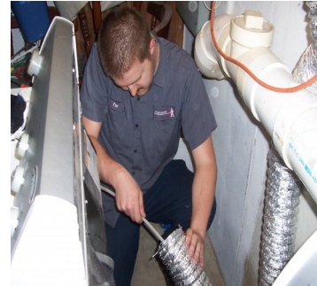
Step12 Dryer vent Cleaning after air ducts
