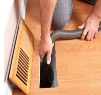
Step9 Vacuum behind brush to clean out debris
