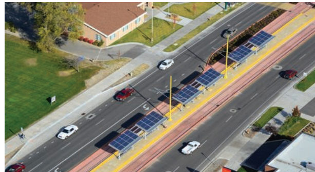
Figure 3-2. Green Line TRAX Station with Rooftop Solar
