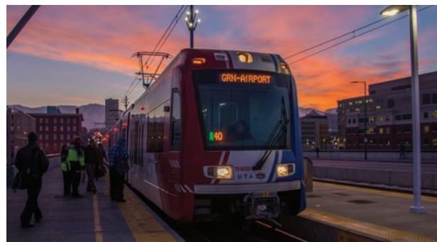
Guadalupe TRAX Station, which connects LRT, commuter rail, bus routes and micromobility with a densifying mixed-use neighborhood, is an example of the sustainable multimodal connections that Research Park is seeking to create.
