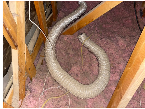
Terminates in attic
