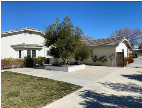
Left side of the home
