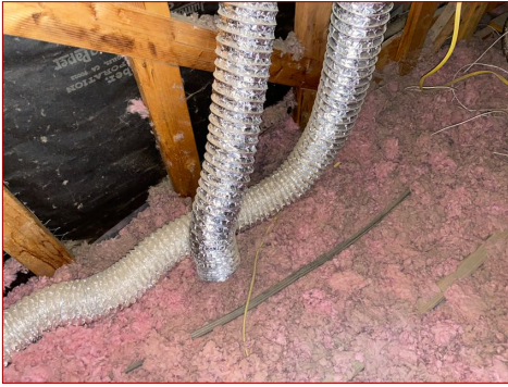
Terminates in attic
