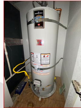
North side of home
