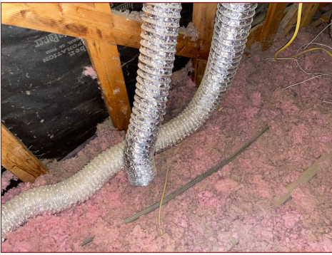
Terminates in attic
