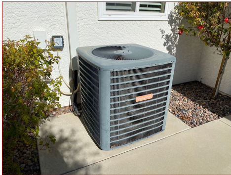
South side unit
