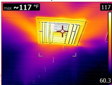
117 degrees - South side of home
