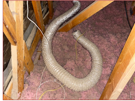
Terminates in attic
