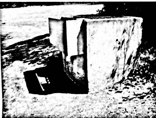
Fig. 5 The control structure for Pond 3
