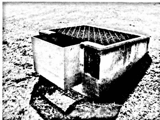
Fig. 6 The control structure for Pond 4
