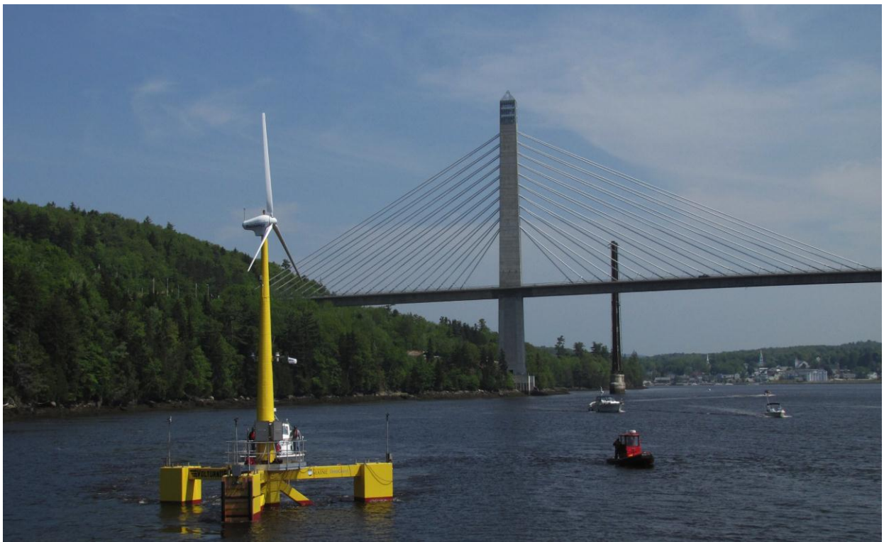
Figure B-2. VolturnUS Floating Turbine
