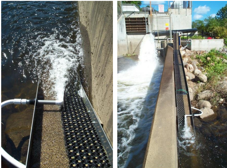
Figure 1. Eel Ramp Example (source CTDEEP)
