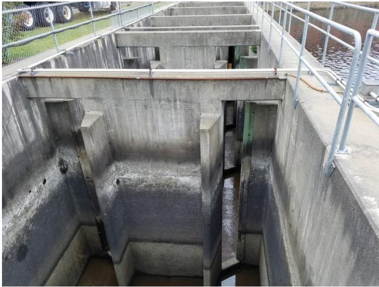
Figure 5. Double Vertical Slot Ladder Example
