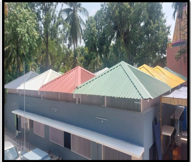
PYRAMID ROOF OF THE BUILDING
