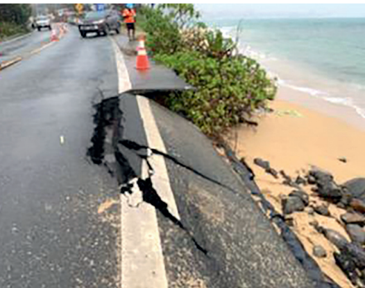
A section of Kamehameha Highway collapsed last year in Hauula due to wave runup.
