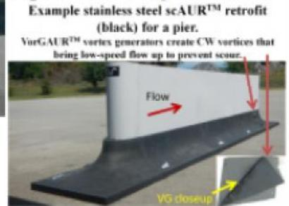
Example stainless steel scAUR™ retrofit (black) for a pier. VorGAUR™ vortex generators create CW vortices that bring low-speed flow up to prevent scour.
