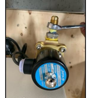
3. USING A WRENCH CAREFULLY TIGHTEN BRASS UNION TO THE SOLENOID OPENING. FIRMLY HOLD SOLENOID SO AS NOT TO ALLOW IT TO TURN
