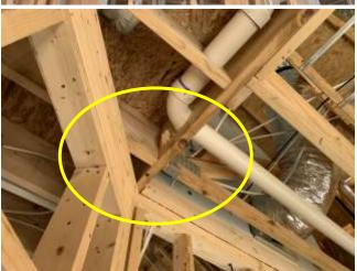
6. Support beam at rear bedroom entrance on first floor has been cut and damaged for plumbing pass-through and the nails from a truss plate. Recommend evaluation by builder to determine if this is causing a weight load deficiency at this location.
