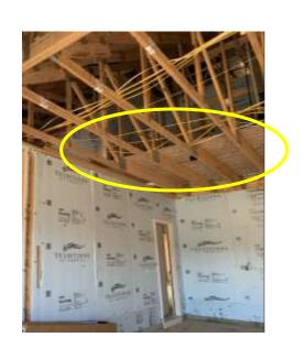
7. Utility room is located above the garage which carries substantial weight load from appliances and potential storage. The floor support is dimensional wood conjoined with roof trusses with metal plates in the ceiling of the garage. The trusses are plated to the rafter chord for support at the top. Recommend final evaluation by the builder and/or an engineer to determine if this is adequate support for a finished utility room
