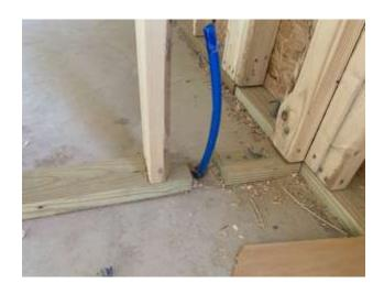
5. Missing kickplates at pex water line to refrigerator. Recommend installation to prevent errant nail or screw puncturing piping
