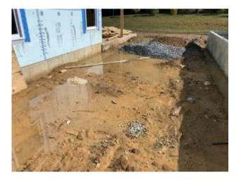
2. Considerable water pooling was noted on the southside yard. Confirm with builder for drainage and grading to draw water away from the structure.
