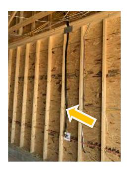
4. Gas line in garage wall has protective plates at the header. Consult with builder if any protections are installed for the vertical length of the gas line as an errant nail or screw that may miss the stud while installing hooks or brackets on the garage wall can still puncture the line.
