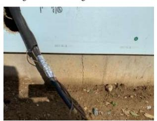
1. Hairline crack is noted in the foundation on the south side wall near the AC refrigerant line. Consult with builder if an epoxy sealant will be applied.
