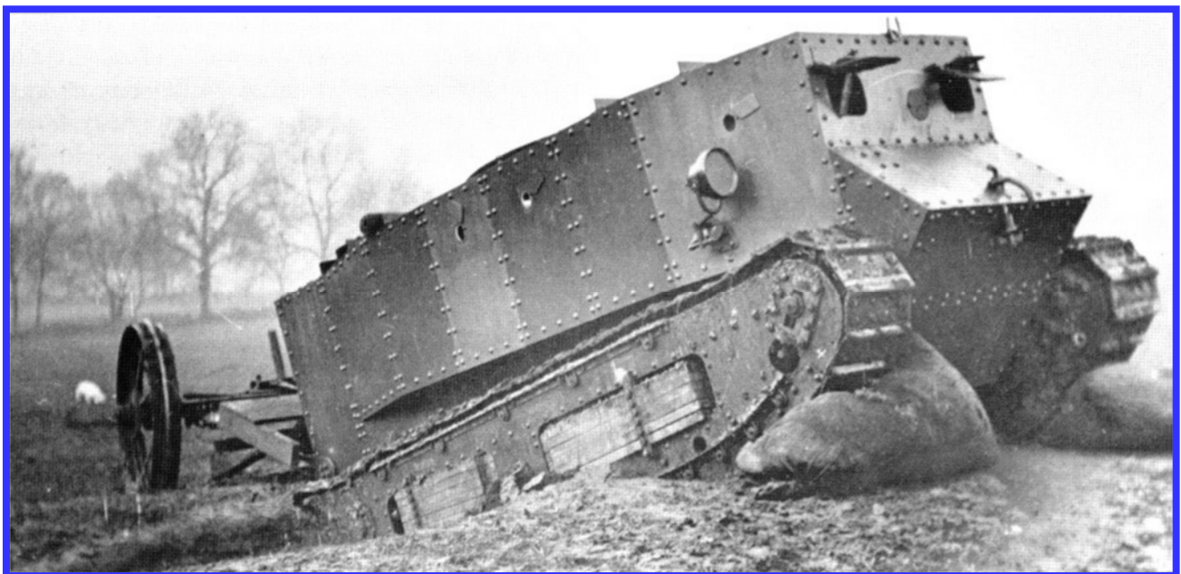
"Little Willie" British prototype of the first tank
