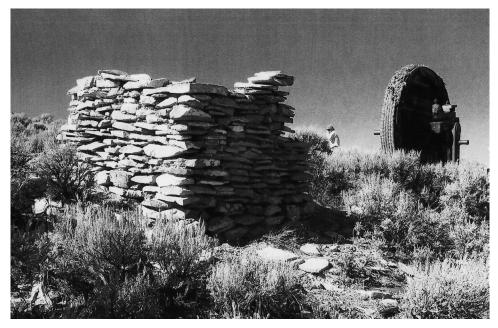
Figure 13: Stone platform possibly to support a steam boiler with a bull wheel shown in the background between the McNaughton #9 and #10 wells.
