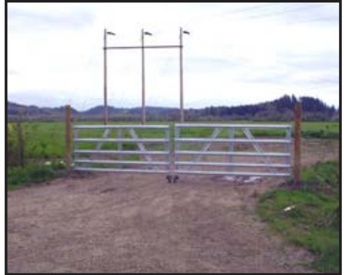
Recently installed gate at the main site access
