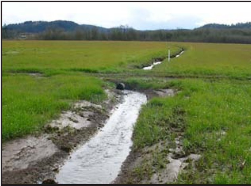
Culverted crossing of Coyote Swale
